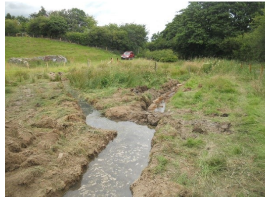
Existing channel plugged. Flow diverted to side channel and new pool. Silt mats placed in old channel to trap disturbed sediment.
