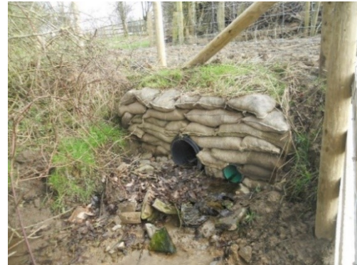
Outfall into field ditch, protected by bagged headwall and new fences.
