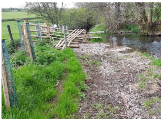
Drinking bay damaged by flood debris.
