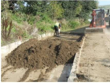
Site preparation: clearing the catchpit, swale & trackside of accumulated sediment
