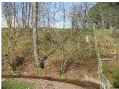
AFTER. Steep bank fenced, to improve stability through regenerating tree and shrub cover.
