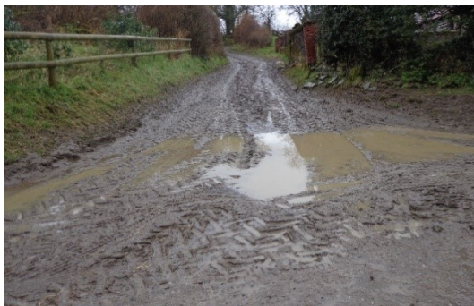
Farm track showing sediment laden runoff being carried onto road.
