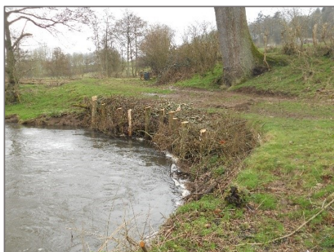
2019. Live willow revetment installed.
