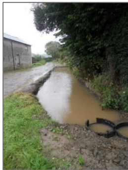
Swale at capacity
