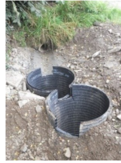
Periscope type outlet connected to pipe outlet by concrete channel
