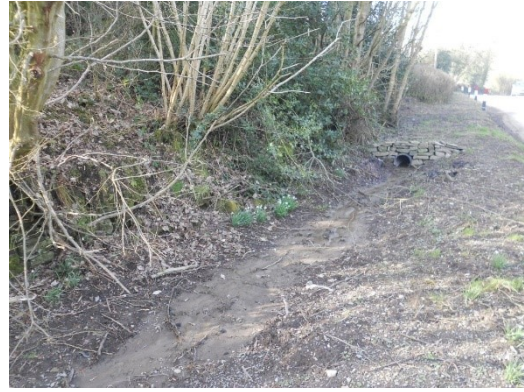
Pipe installed and outfall protected with stone headwall.
