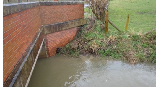
Pipe outfall to river, showing silt plume
