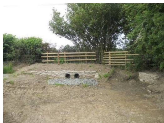
New outfall with headwall completed & backfilled. July 2020.
