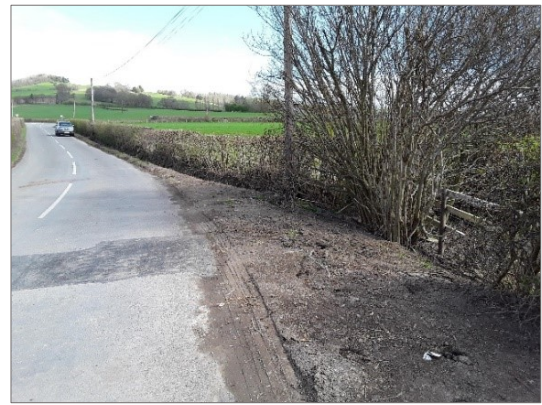
Roadside ditch carrying road runoff to new swale. July 2020.
