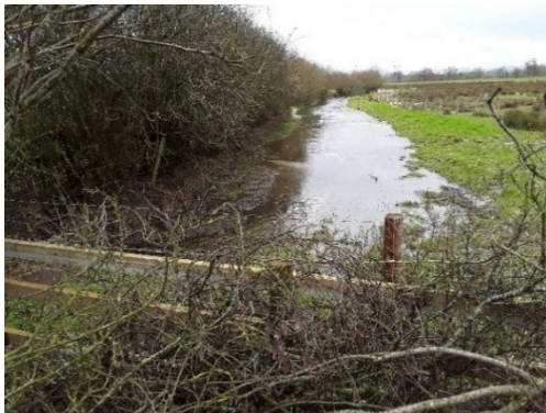
Functioning swale close to capacity. February 2021.
