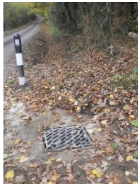
Grid covered catchpit & sump, receiving runoff from restored roadside ditch.
