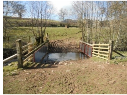
AFTER. New fencing and made-to-measure river gates installed.
