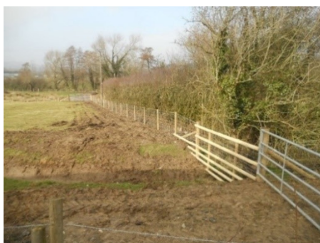
Ditch protected by stockproof fence. Gated access to adjacent field over pipe culvert.
