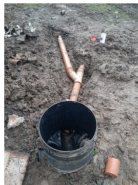
Existing pipe connected to new catchpit
