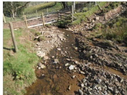
Stock & vehicle crossing point now closed off, limiting gully erosion on bank.
