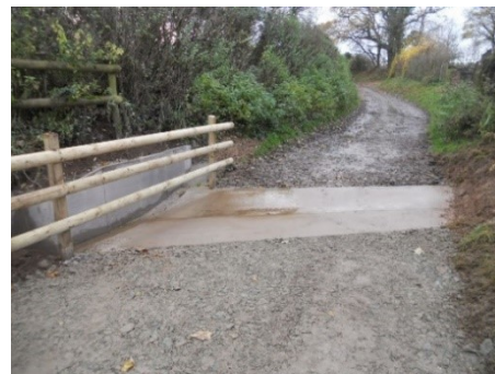
Concrete dish cross drain built in situ to intercept track runoff.
