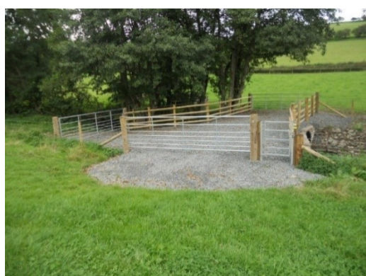
AFTER. View from right bank. Culvert installed, fenced & gated, plus pedestrian gate on PRow.
