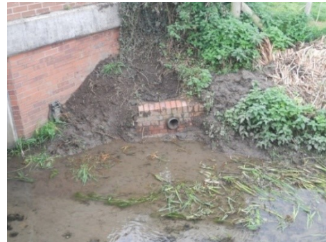
Outfall to river with new brick headwall
