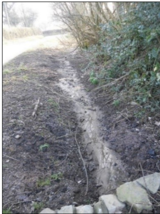
Open ditch from outfall showing silt settling out from the runoff.
