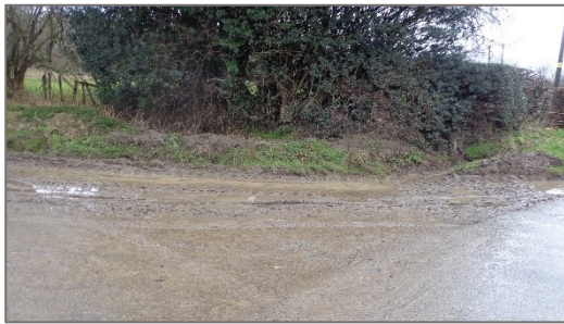
Runoff flowing onto highway and ditch
