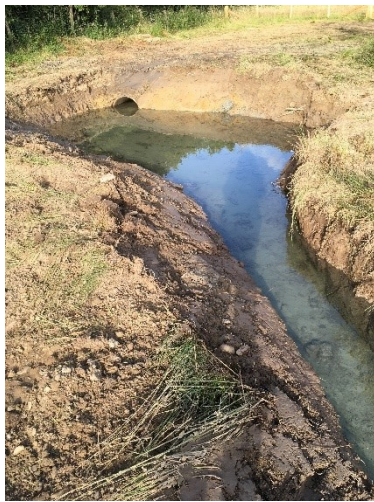
New outfall after pipe removal. Large pool created to minimise impact during high flow.
