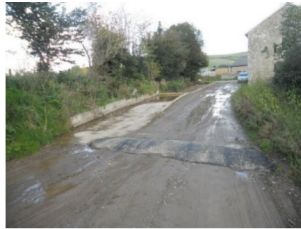
Tarmac "sleeping policeman" to direct runoff into catchpit
