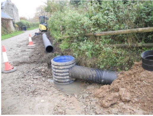
Catchpit with sump showing pipe to be installed along roadside verge.
