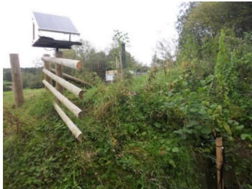
60w solar panel on bespoke frame.
