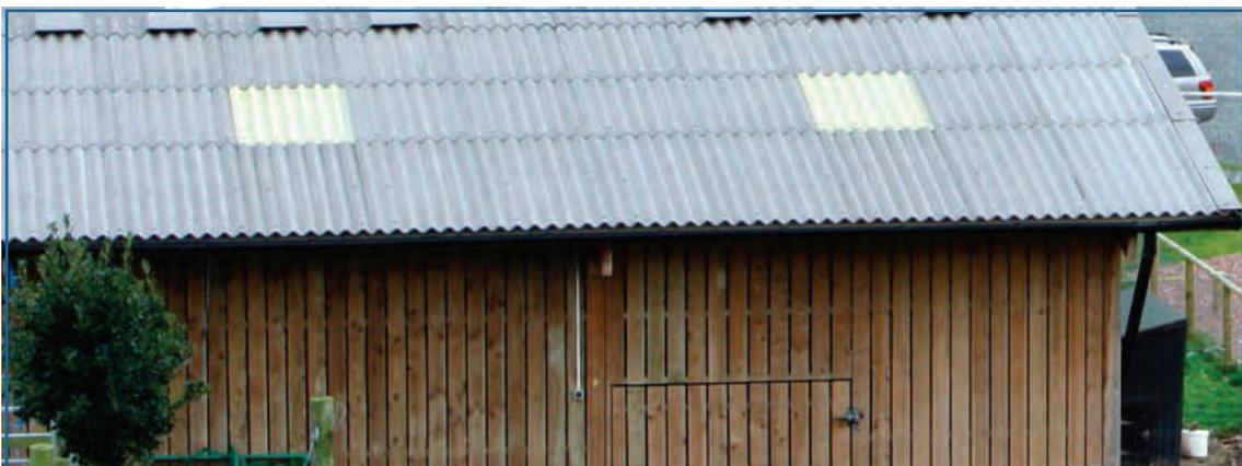
Figure 22: Overlapping Eaves should project to the maximum
