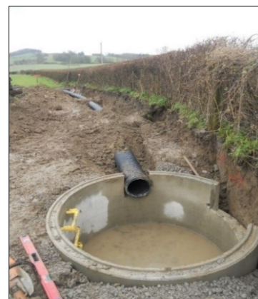
Catchpit with new supply pipe installed
