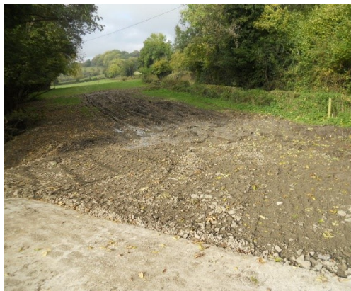
BEFORE: Rutting and compaction created during bridge installation
