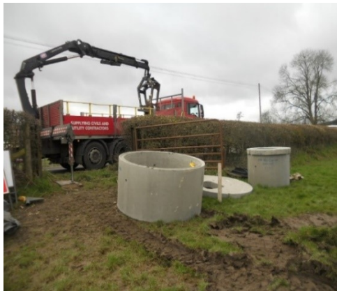
Delivery of concrete catchpits
