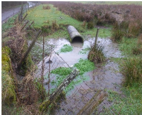
Outfall into pool. Shows colouration from sediment laden run-off
