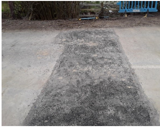
Road crossing completed, with tarmac covering
