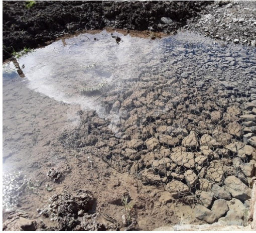
Headwall with gabion mattress apron for erosion control
