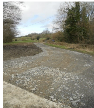
AFTER: Roadside gate realigned, to meet reggraded track with new stone surface.
