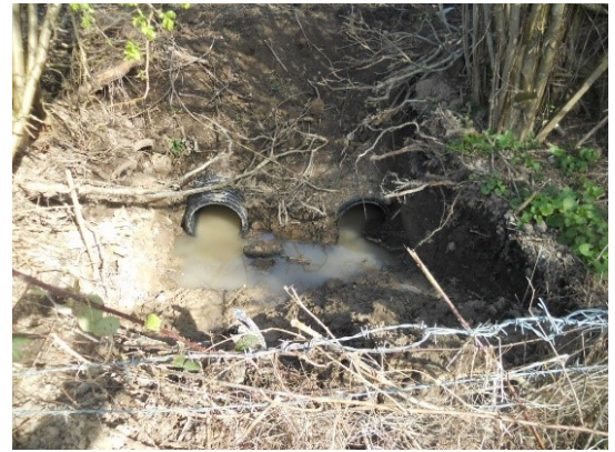
New culvert, showing temporary outfall
