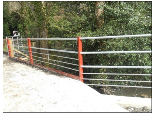
AFTER: Additional rails installed to make stockproof for sheep & lambs
