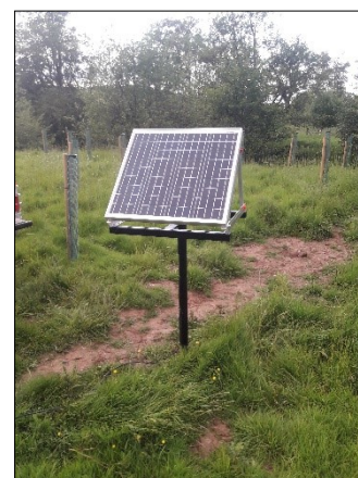
60w panel mounted on homemade frame
