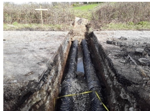
Culverted road crossing showing two 300mm twin wall pipes
