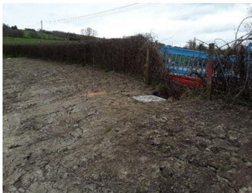
Catchpit with manhole cover and new pipe backfilled and covered with soil.
