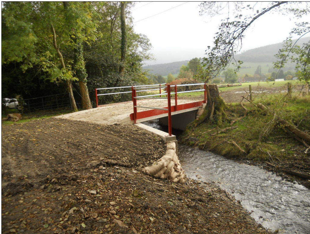
Bridge installed over Clunton Brook to replace livestock and vehicle crossing.
