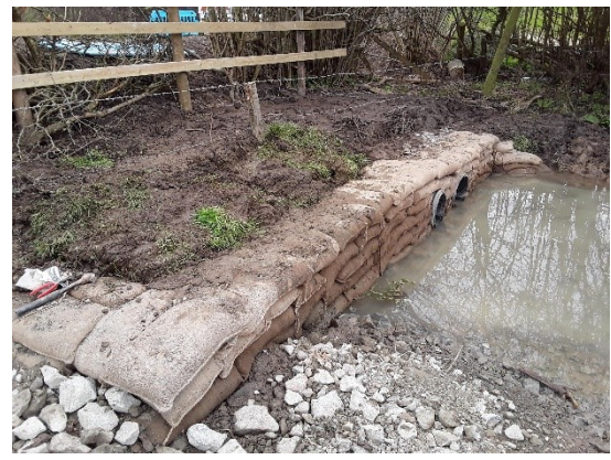
New outfall with headwall completed
