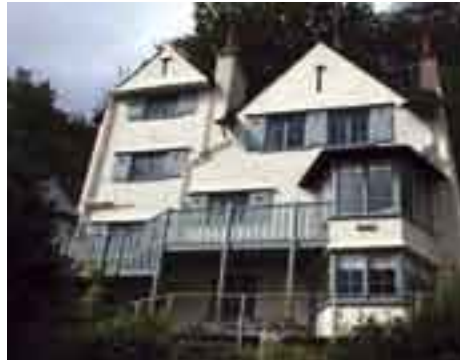
Beam House Madeira Walk
