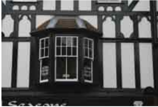
The replacement window on the right does not respect the original character of the building
