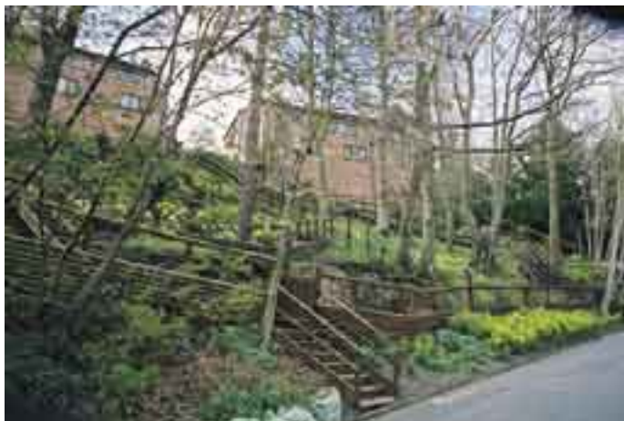
Houses on steep bank, Cunnery Road
