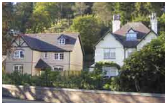
New house and original Edwardian house
